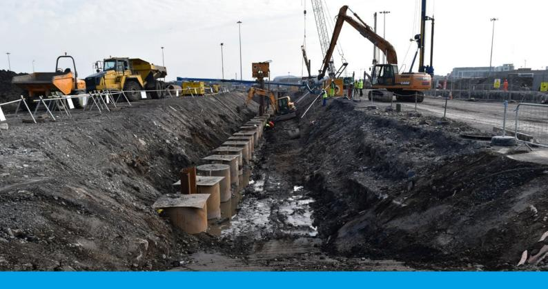
THE ALEXANDRA BASIN REDEVELOPMENT INVOLVES THE CONSTRUCTION OF APPROXIMATELY 3KM OF QUAY WALLS, DEEPENING OF THE HARBOUR BASIN AND CHANNEL TO ACCOMMODATE LARGER SEA GOING VESSELS AS WELL AS WORKS ASSOCIATED WITH THE CONSERVATION OF THE PORT'S VICTORIAN INDUSTRIAL HERITAGE.
