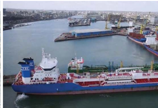
ALEXANDRA QUAY EAST
