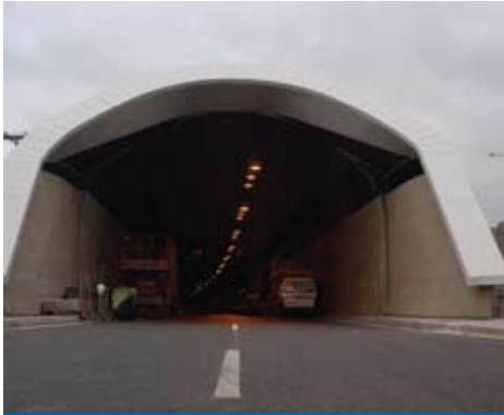
Dublin Port Tunnel
