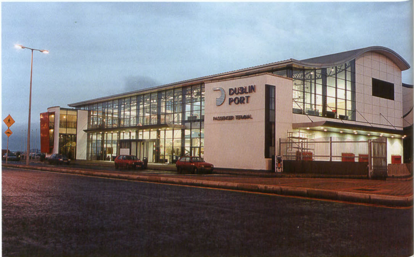
Passenger Terminal No.1
